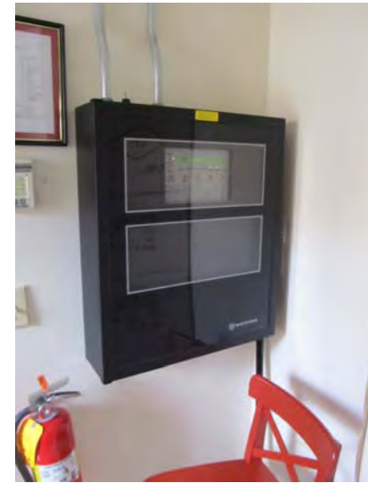
Fire alarm system upgraded in recent years and includes a fully addressable control panel
