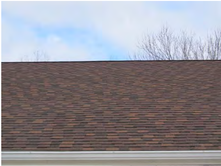
Roof coverings on all buildings recently replaced – No problems noted
