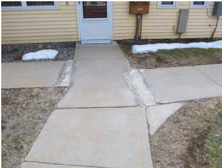
Concrete walkway surfaces in need of repair/sectional replacement at isolated locations
