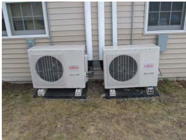
Exterior condensers for recently installed heat pump systems at each apartment
