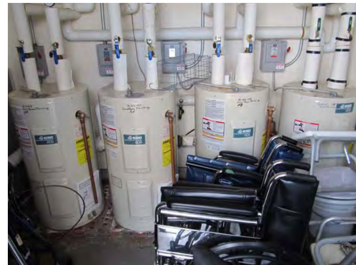
Typical unit-level electric domestic hot water tanks
